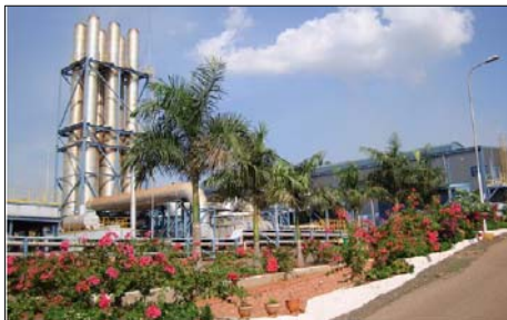
Power Plant III, 6 x 17MW
