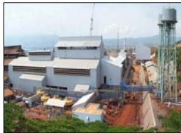
FeNi III smelter complex
