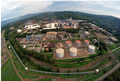
Pomalaa Ferronickel Plant
