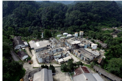
Pongkor Gold Processing Plant
