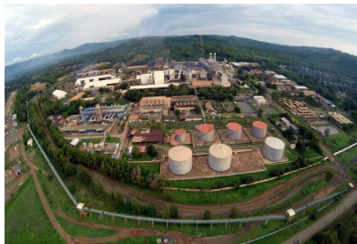
Pomalaa Ferronickel Plant
