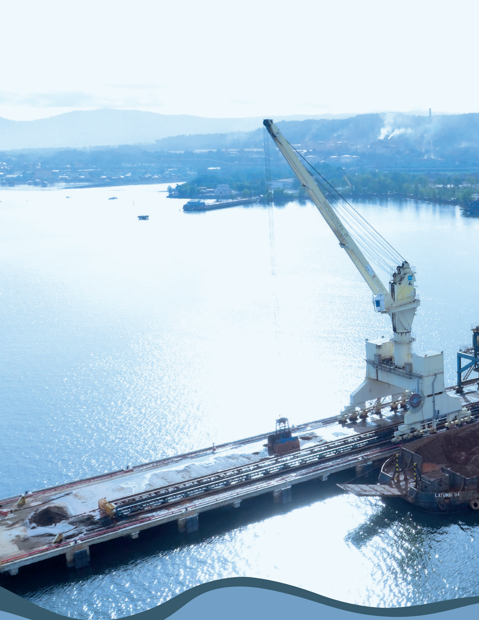
>> Fasilitas Jetty dan Belt Conveyor ANTAM di Pomalaa. ANTAM's Jetty and Belt Conveyor Facility in Pomalaa.
