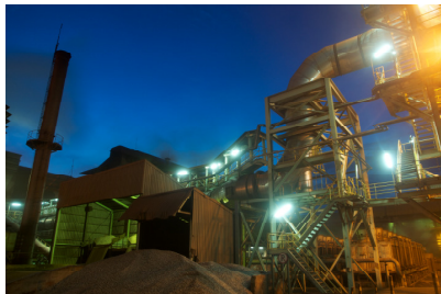
Pomalaa Ferronickel Plant
