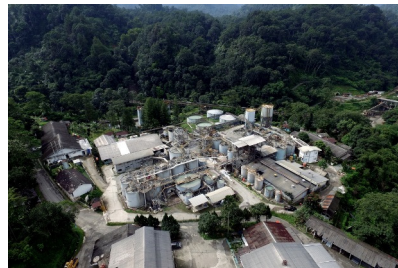
Pongkor Gold Processing Plant
